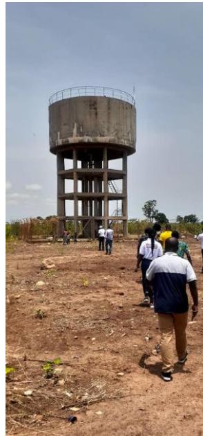
Figure 2 Existing Water Tower in the Oti Region
